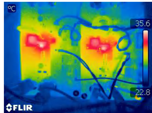
Figure 4-20. Thermal Condition in Dual Phase Boost ( V_{IN}=12V and 2A Load)
