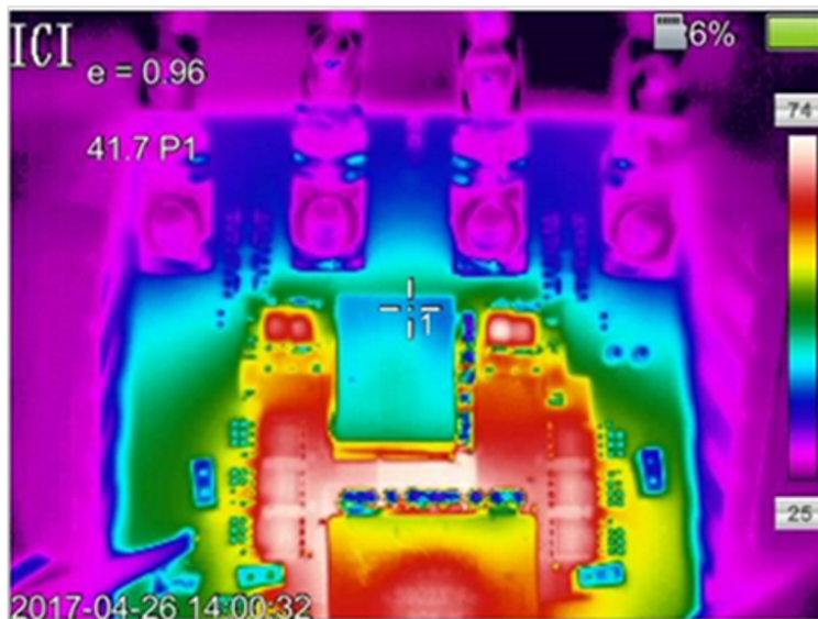
図 37. Thermal Image of Output Inductor (L1)
